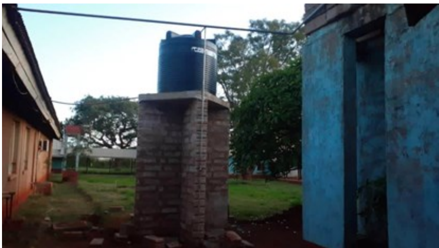
Completed water tower
