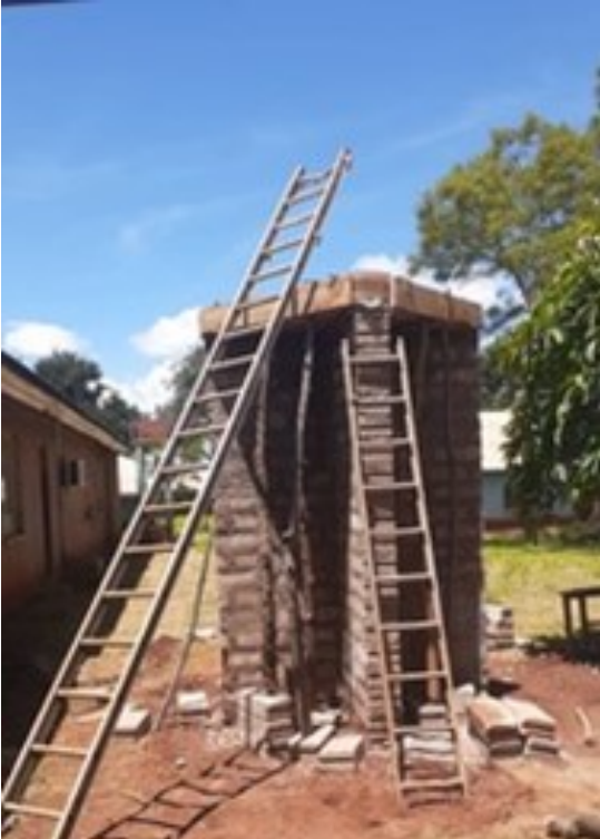
Water platform is built with handmade bricks
