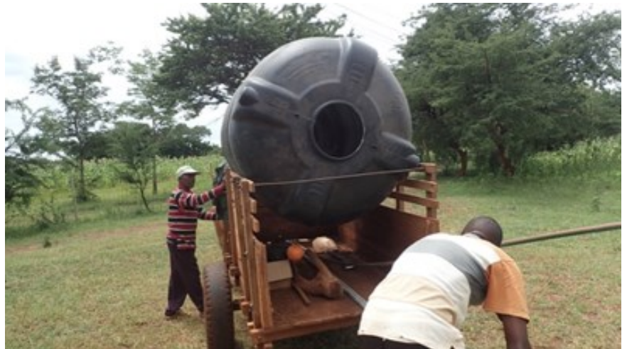
Water tank is delivered to construction site by ox-drawn cart
